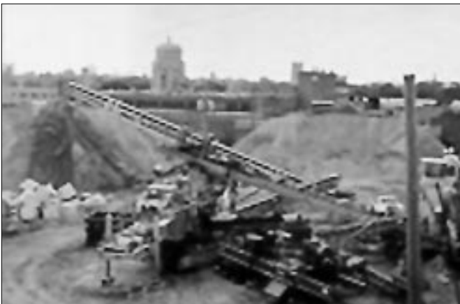
Sacramento Crushing Site Source: City of Chicago
