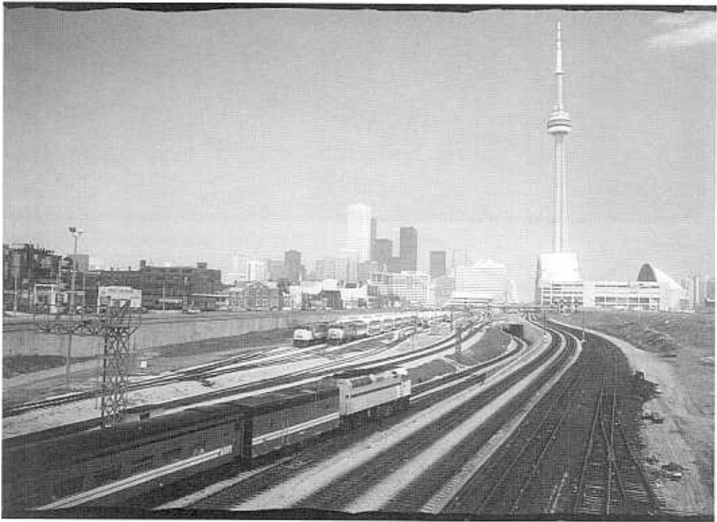
Rail passenger access to downtown Toronto
