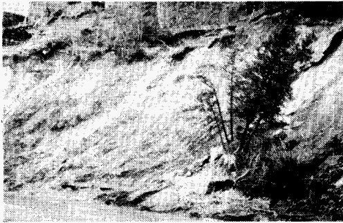
Before stream bank restoration
