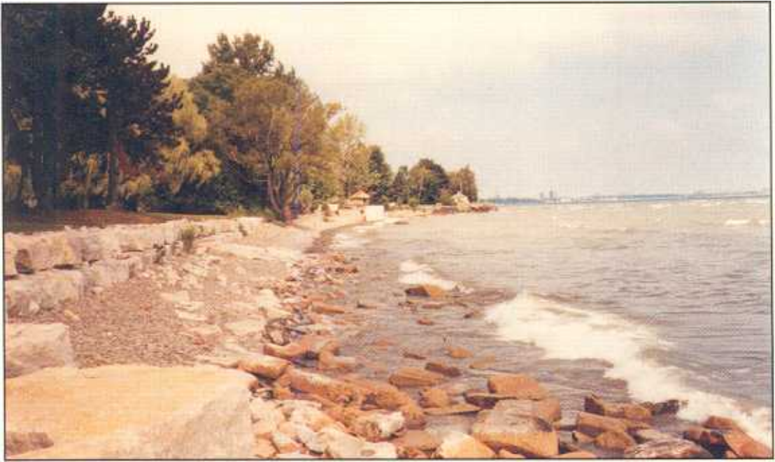
Watersedge Park, Mississauga
