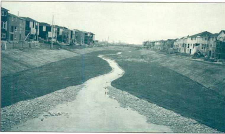
Cooksville Creek, Mississauga: damaged by development practices, this channel is now under restoration by the Credit Valley Conservation Authority and the City of Mississauga
