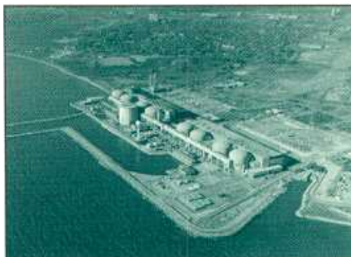
Pickering Nuclear Power Station
